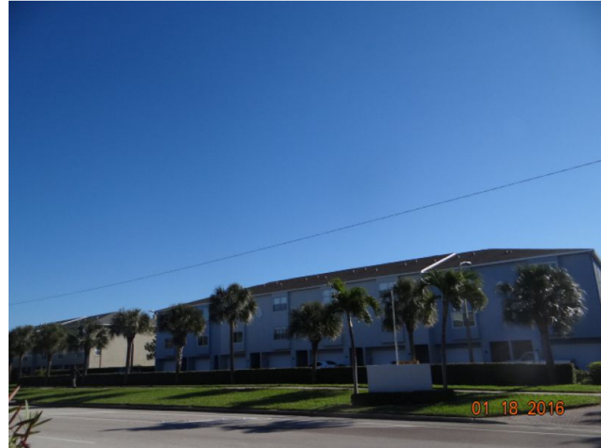
Asphalt/Fiberglass Shingle Roof Covering
