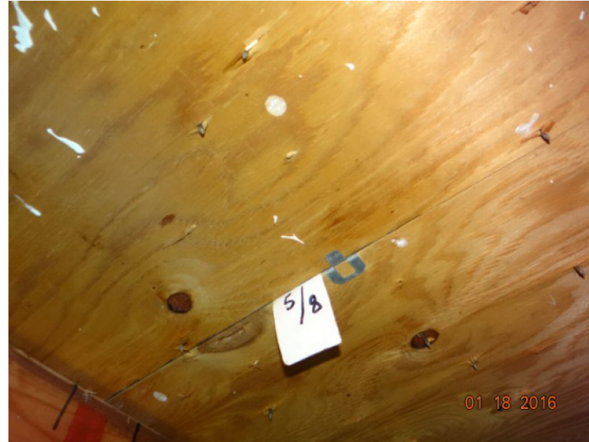
5/8" Deck Thickness Confirmed
