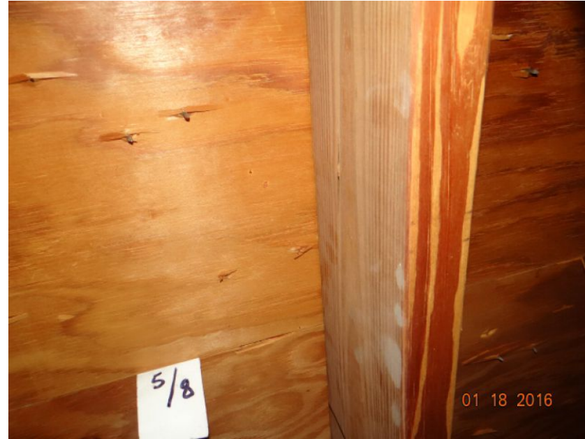
5/8" Deck Thickness Confirmed
