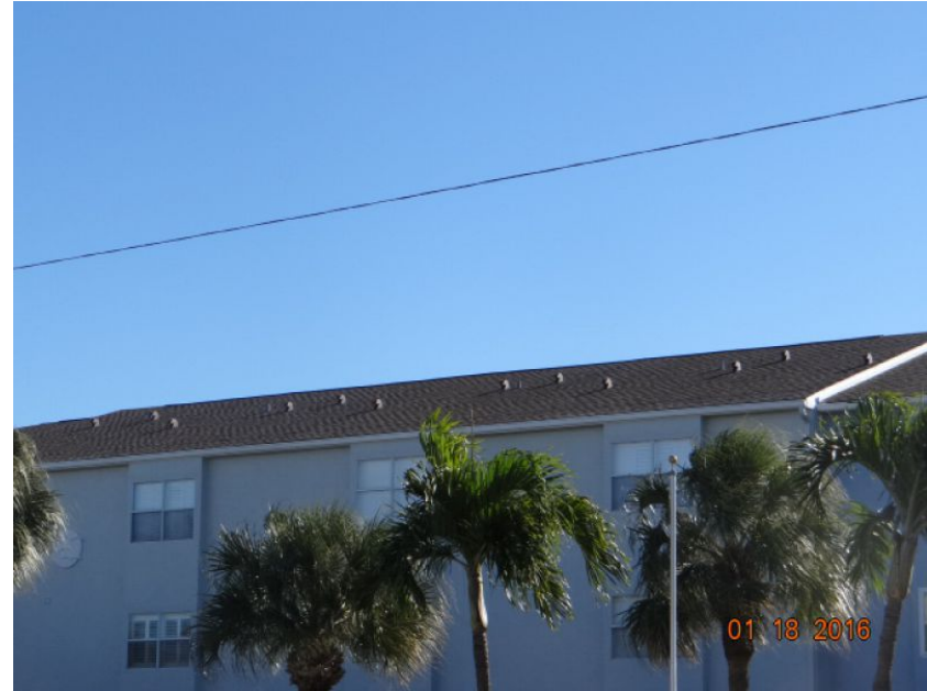
Asphalt/Fiberglass Shingle Roof Covering
