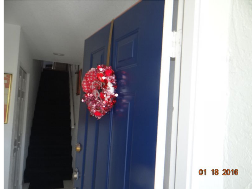
Unprotected Solid Entry Door
