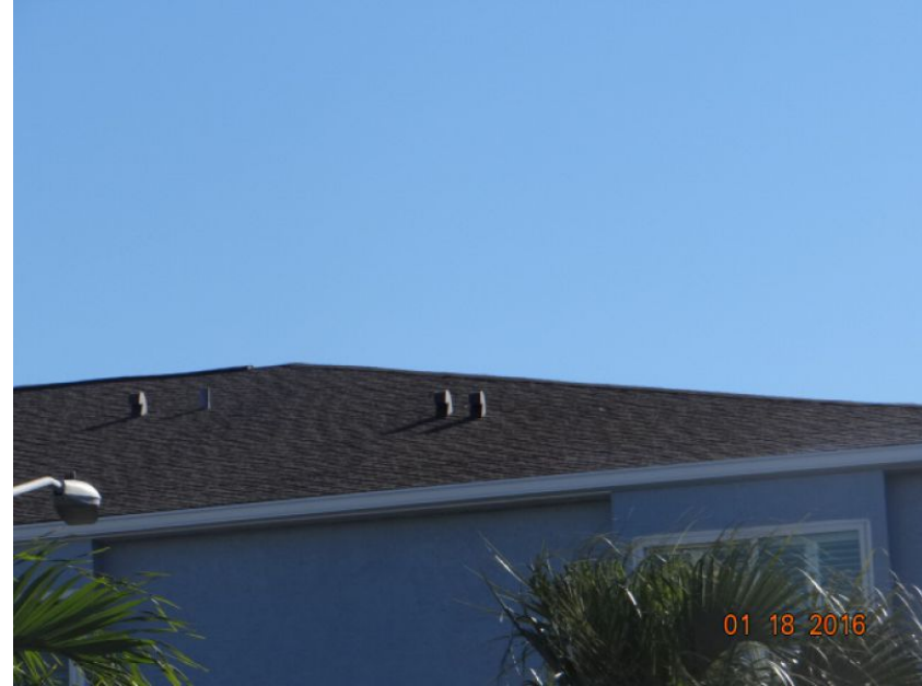
Asphalt/Fiberglass Shingle Roof Covering
