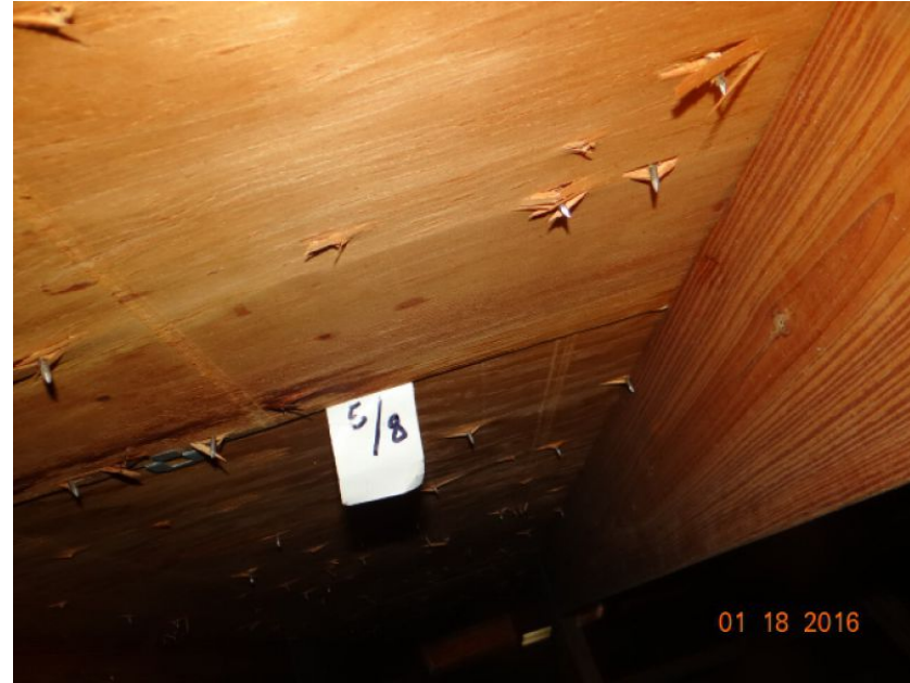
5/8" Deck Thickness Confirmed
