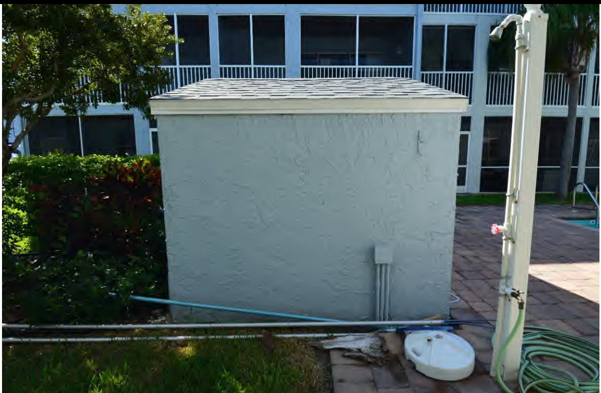
VIEW OF PUMP HOUSE
