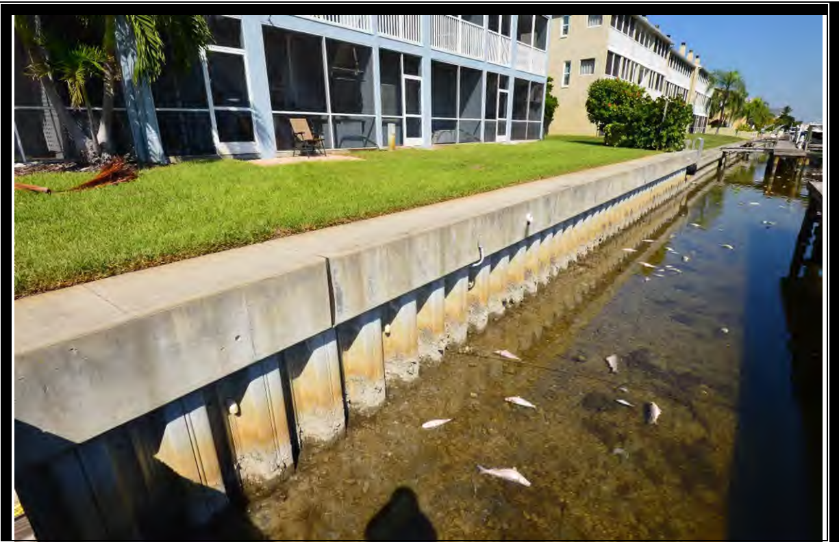
VIEW OF SEAWALL
