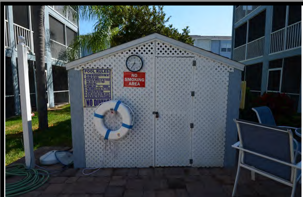
VIEW OF PUMP HOUSE
