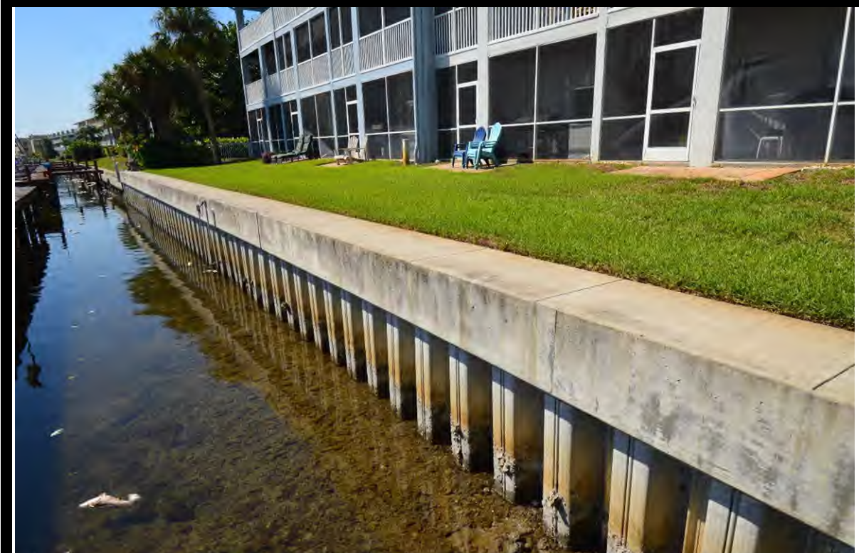
VIEW OF SEAWALL
