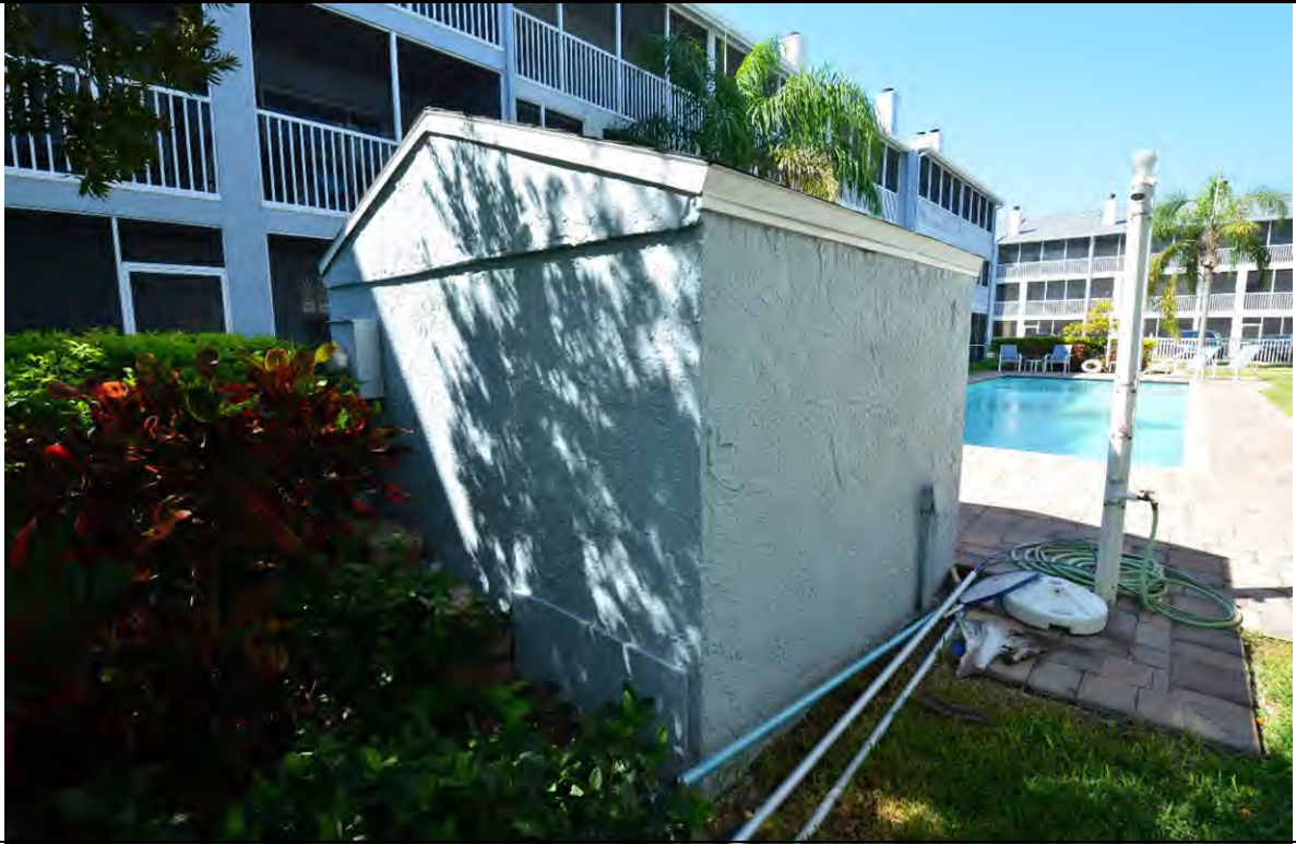
VIEW OF PUMP HOUSE
